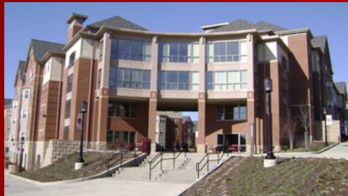
Indiana University of Pennsylvania New Student Housing Complex
