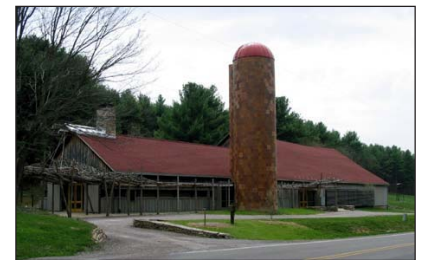
WESTERN PENNSYLVANIA CONSERVANCY MILL RUN, PENNSYLVANIA REGIONAL INTERPRETIVE CENTER AT BEAR RUN NATURE PRESERVE
